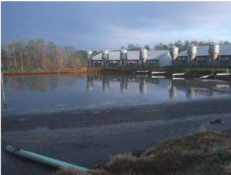
State-of-the-art lagoon waste management system for a 900-head hog farm. The facility is completely automated and temperature controlled (NRCS Photo Gallery NRCSGA02035)
