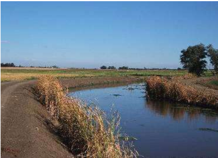
A tailwater recovery ditch near a rice field in northern California (NRCS Photo Gallery NRCSCA02115)
