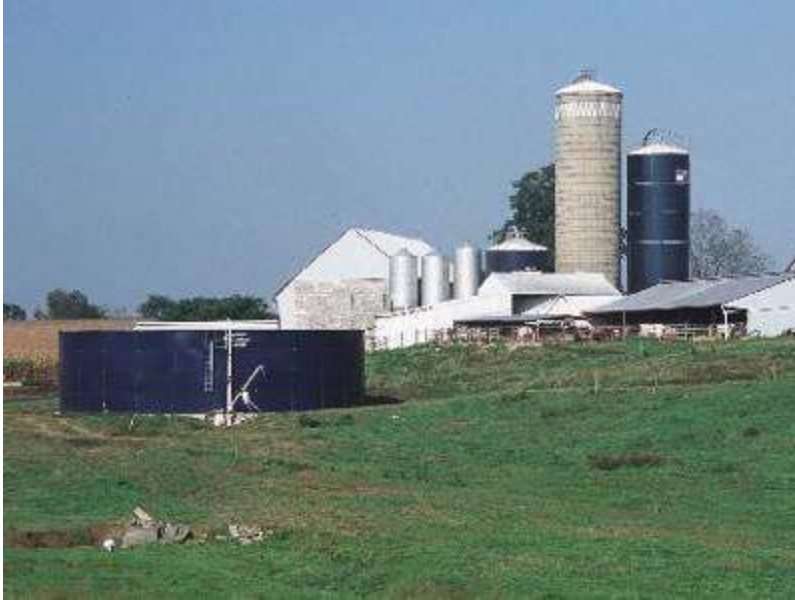
A manure storage tank (part of a conservation plan) on a dairy farm in Lancaster County, Pennsylvania (NRCS Photo Gallery NRCSPA00020)
