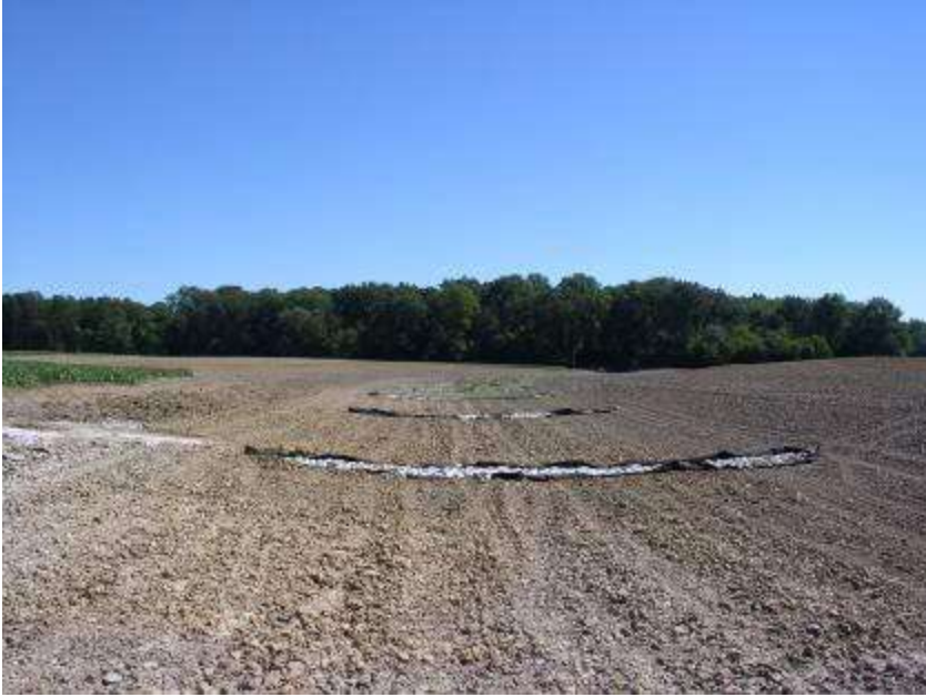
Rock checks installed to reduce runoff velocity in a waterway in St. Clair County, Illinois (Office photo StC1000)
